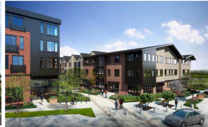
BUILDING B1 & B2 LOOKING NW
