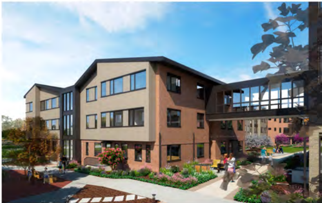
BUILDING B1 & B2 LOOKING NE
