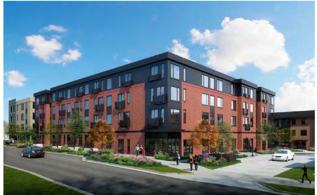
BUILDING D LOOKING NW
