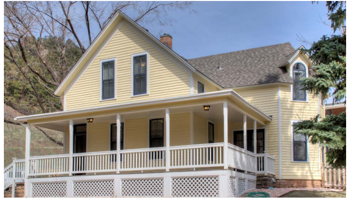
Cornell House: 1 Unit Full historic renovation.
