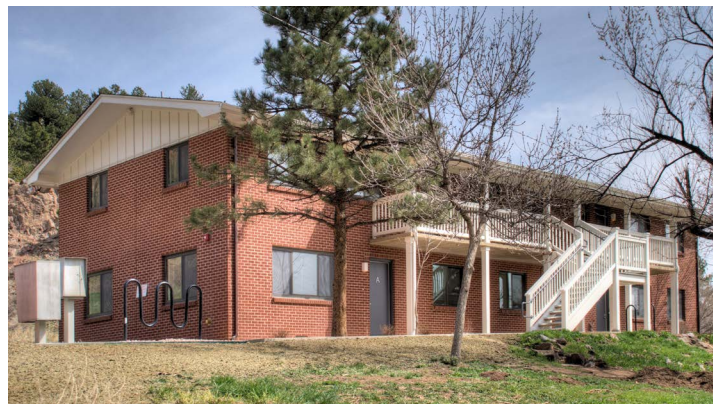
The Flats@101 Canyon: 5 Units Comprehensive market rate renovation.
