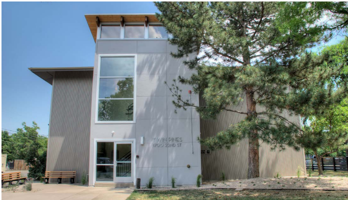
Twin Pines: 22 Units Comprehensive interior, exterior and site renovation.
