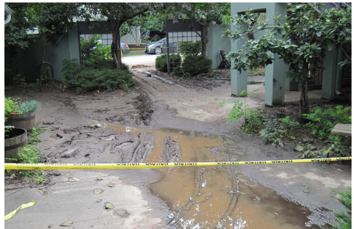
Flooded courtyard at Arapahoe Court.
