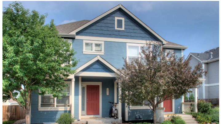
Dakota Ridge: 13 Units. Exterior paint, hot water tanks, flooring, storage units, landscaping.
