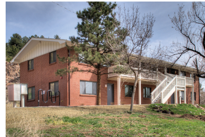
The Flats @ 101 After
