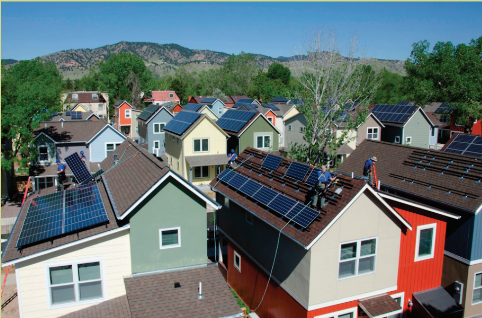
Red Oak Park Solar Installation
