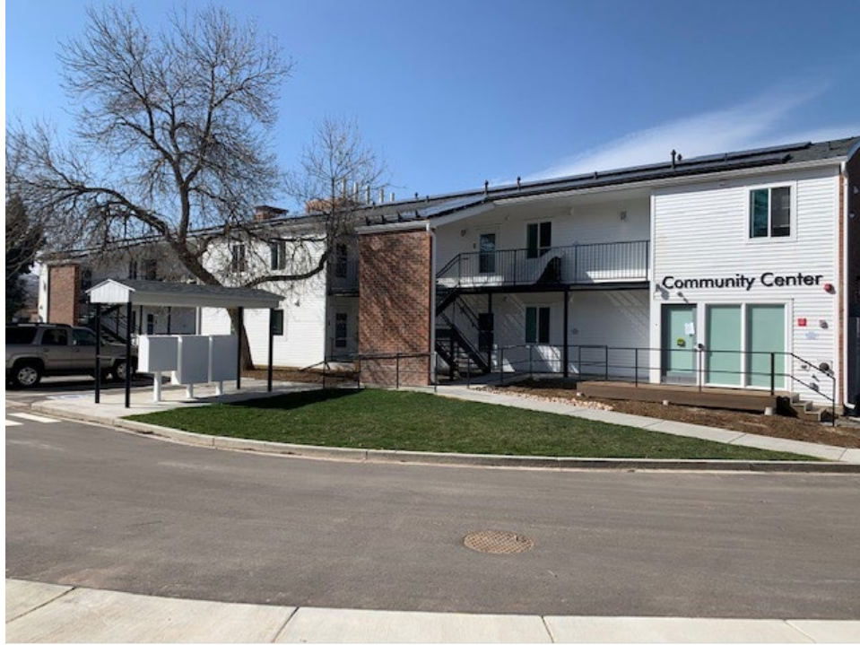
Renovated exterior of Madison Apartments.
