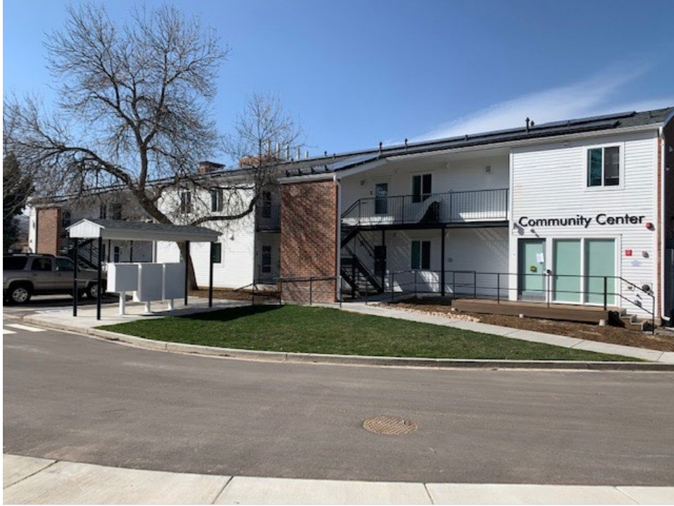
Renovated exterior of Madison Apartments.
